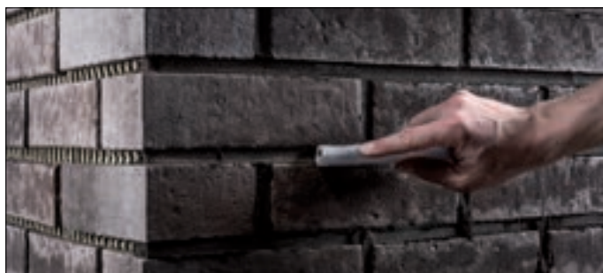
Trowel jointing can be used to create different looks.
